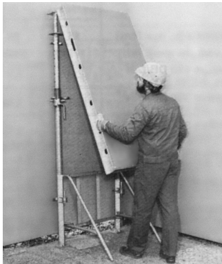
Step 3 Fit Panel onto lugs on the Bearing.
