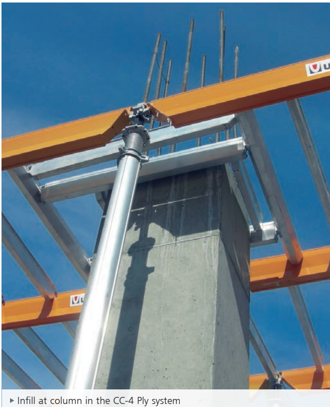
► Infill at column in the CC-4 Panel system
