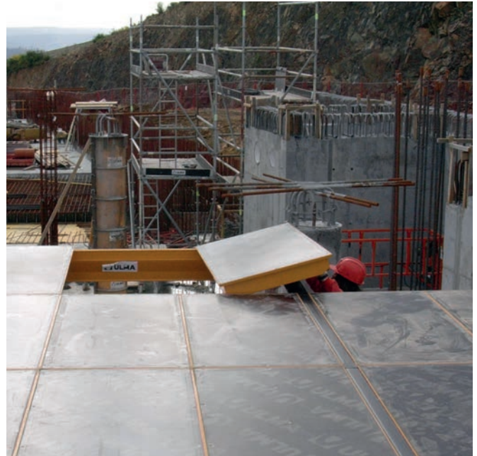
► Easy assembly by sliding the panels into place
