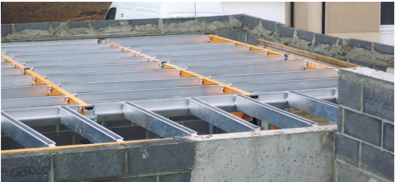
► Infill at wall in the CC-4 Ply system
