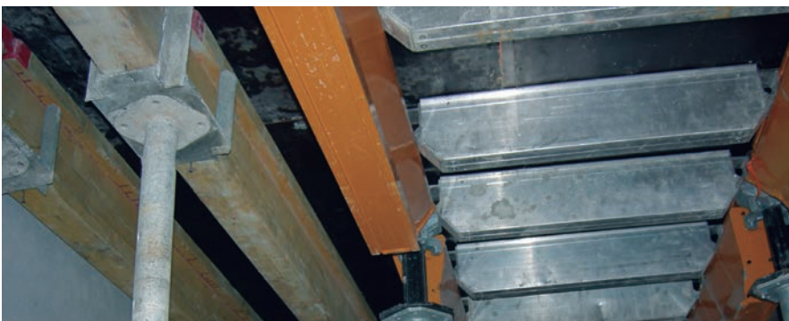
► Beams VM on props that provide support for the infill plywood
