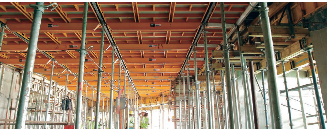
► Shuttering face with phenolic plywood or composite board
