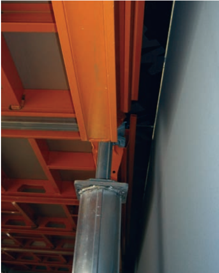
► Infills at walls with edge beam as infill plywood support
