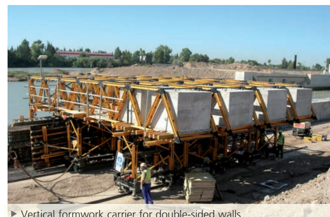
► Vertical formwork carrier for double-sided walls
