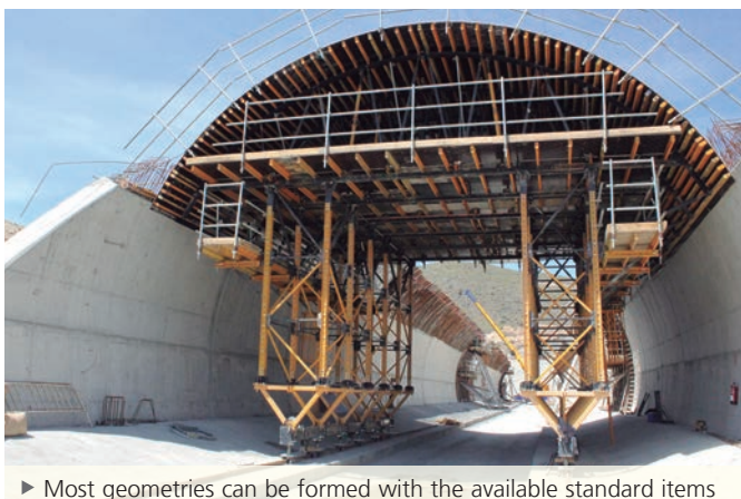
► Cut-and-cover tunnel
