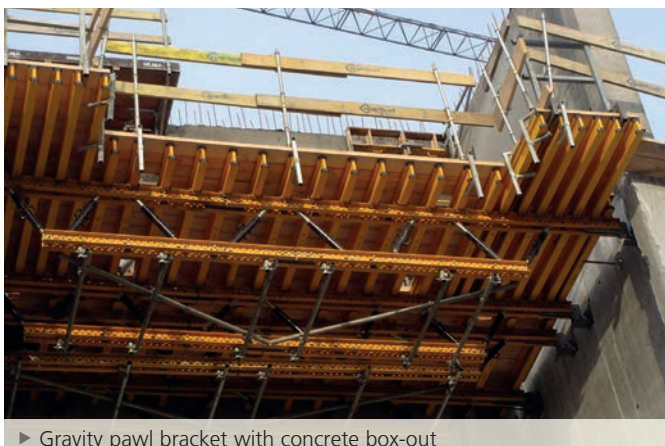
▶ Gravity pawl bracket with concrete box-out
