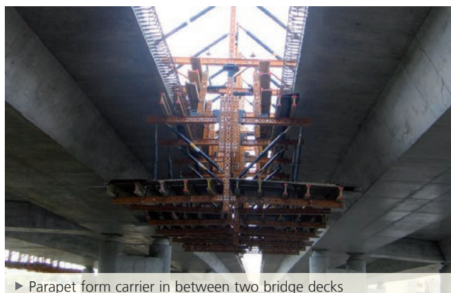
► Parapet form carrier in between two bridge decks
