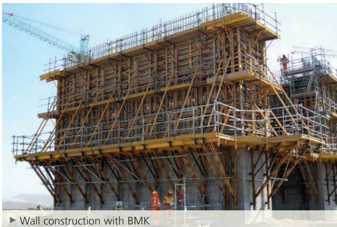
▶ Wall construction with BMK
