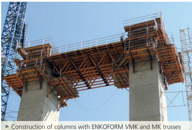
▶ Construction of columns with ENKOFORM VMK and MK trusses
