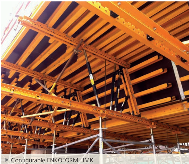
▶ Combination of ENKOFORM HMK and T-60 Shoring
