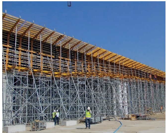
▶ Combination of ENKOFORM HMK and T-60 Shoring
