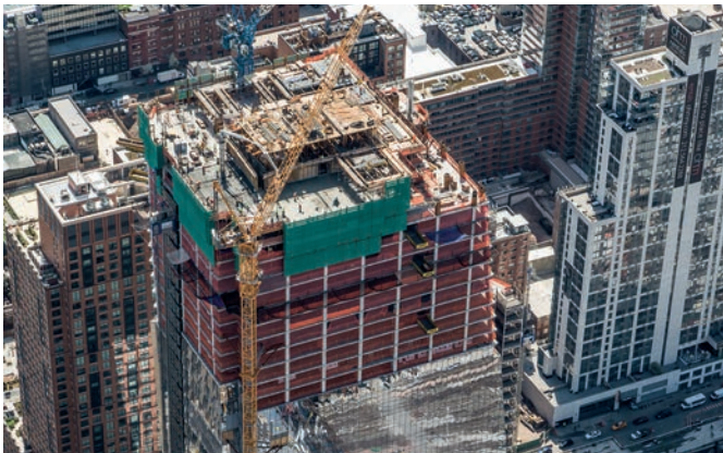
▶ Construction of building core with ATR Self-Climbing system
