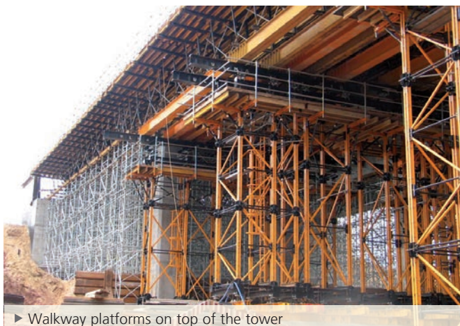
▶ MK shoring used at height
