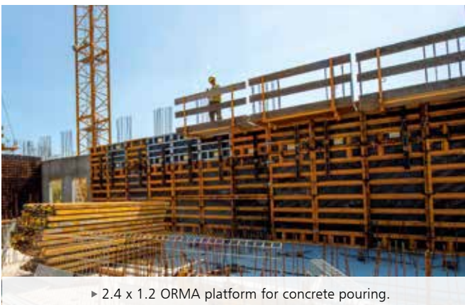
► Working platform with ORMA Walkway Brackets at different levels.
