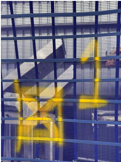
Photograph 3. Detail view of M01- Blue Uni-mesh at point 01 after test.
