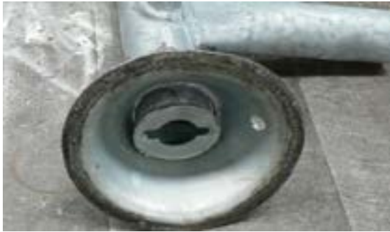
5. Collapsed or missing foot plate.
