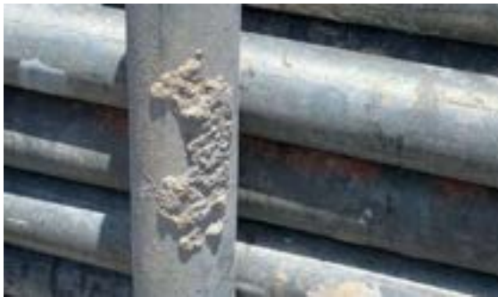
7. Build up of concrete.
