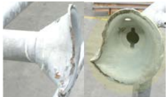
4. Damaged and distorted Foot Plate.
