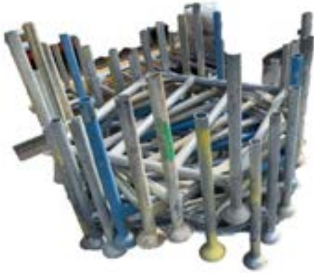
Incorrect way of stacking
